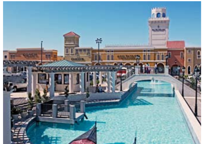
Prime Outlets, San Marcos, TX
